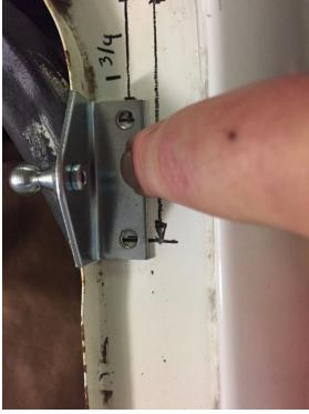
7. Find the proper drill points by using the lower bracket as a template and pressing your pencil INWARD as shown, while dragging the bracket along the standing metal edge.
